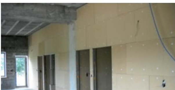
UdiCLIMATE® is applicable as an underside, roof insulation board or dry lining layer for walls
