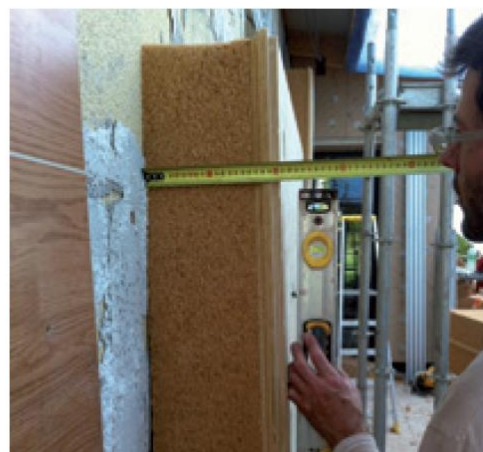
The UdiRECO SYSTEM adapts to the surface to provide a snug, wind-tight fit
