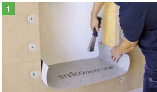
Attachment of STEICO multi UDB (diffusion-open membrane) as temporary weather protection until window installation.
