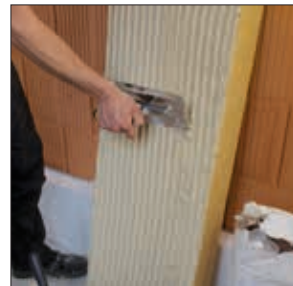
Glue the insulation board to a flat surface with full-surface bonding
