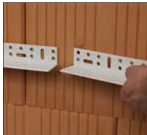
Attach angle rail
