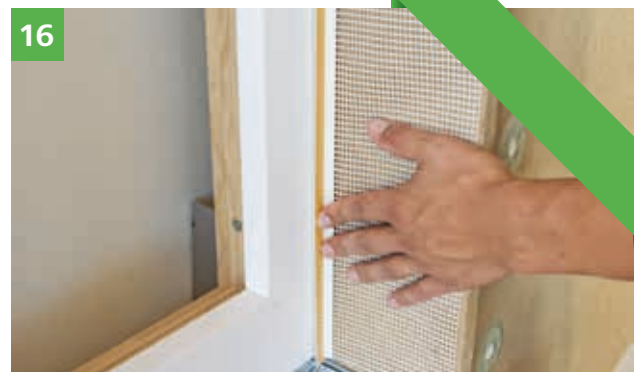
16 Attachment of a suitable rendering strip for safe render termination and continuation of ETICS work.
