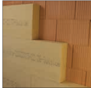
Installation of small-format blunt slabs
