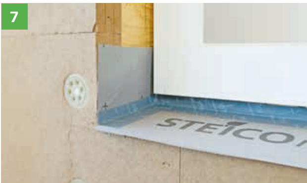
Insert the STEICO fix insulation wedge into the reveal, remove the remaining adhesive tape liner and press on the STEICOmultiply F adhesive tape.
