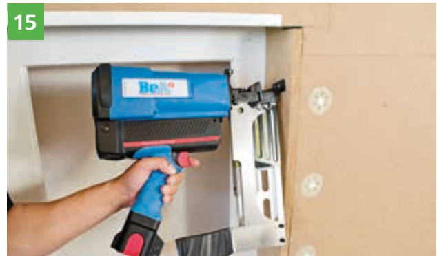
15 Fixation of the reveal board for undisturbed hardening of STEICOm ulti fill by means of wide back clamps or stainless steel screws.
