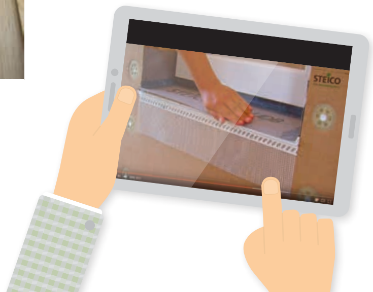
14 Inserting the reveal board flush with the outer edge of the ETICS façade TIP: If necessary, plan for window frame widening.
