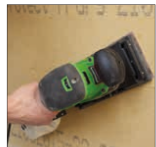
Grinding board offsets
