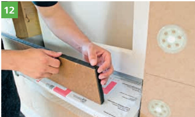
12 Installation of the reveal board. Protection against driving rain by applying joint sealing tapes to the front and end edges.
