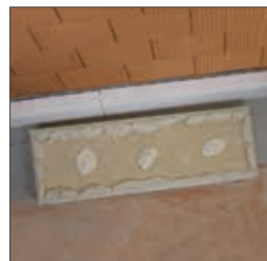
Adhesion of insulation boards on uneven surfaces using the point and bead method
