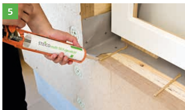
STEICO multi fill adhesive beads are used to secure the insulation wedge against lifting off, e \leq 30 cm.
