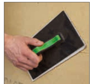
Grinding board offsets
