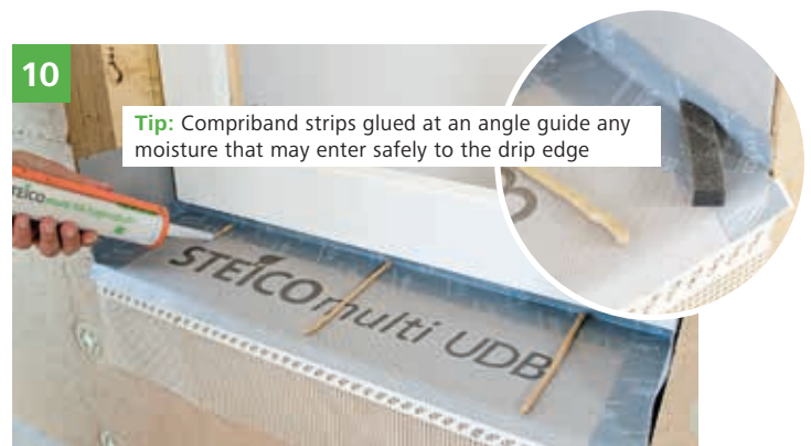
Application of STEICOmultiply adhesive beads e \leq 30 cm for the elastic fixing of the windowsill.
