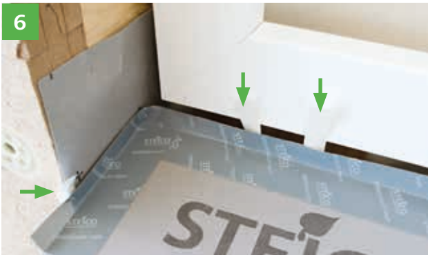
Installation of the STEICO fix insulation wedge. TIP: Fold back release paper, it can be removed more easily later.
