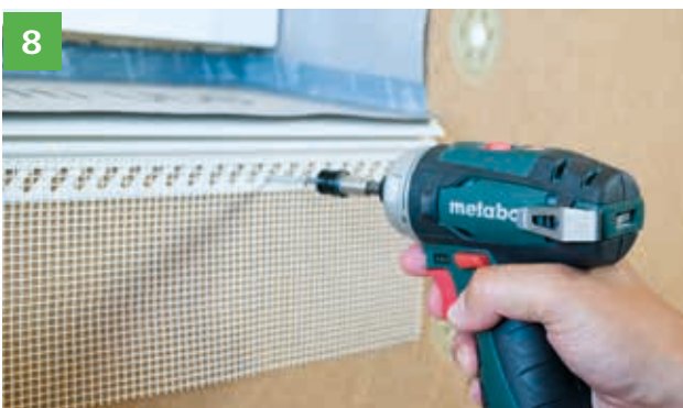
For a secure render connection, an attic profile is installed below the STEICO fix wood fibre insulation wedge (stainless steel screws or clamps in the wood fibre insulation board).
