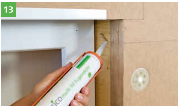
13 Application of STEICOm ulti fill adhesive beads into the wooden frame construction to ensure a secure hold of the reveal board.
