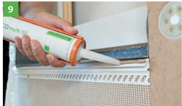
The protruding flap of the laminated underlay is glued to the drip edge of the parapet profile using STEICOmultiply.
