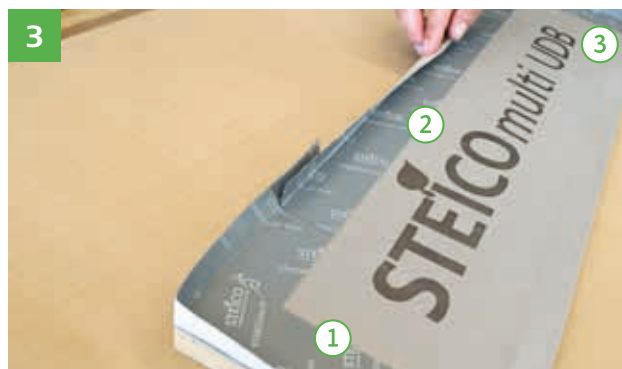
The STEICO multi tape F adhesive strips are then attached to the insulation wedge in such a way that a three-sided "trough" is formed
